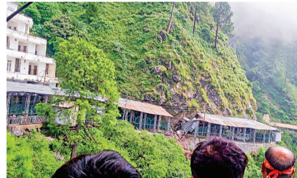
A structure on a track towards the Vaishno Devi shrine got collapsed due to landslide, in Reasi on Monday. ANI
