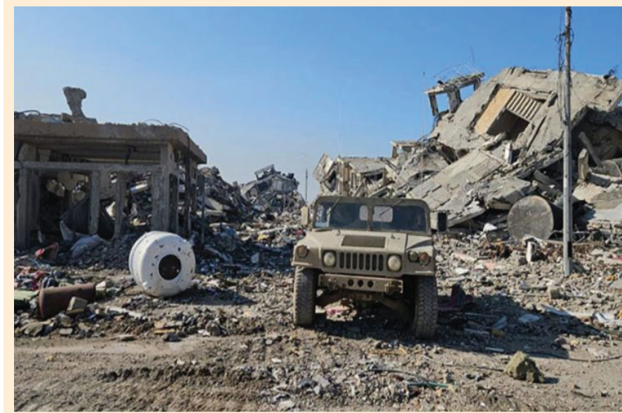
War-torn area and dilapidated buildings in Gaza. File Photo
