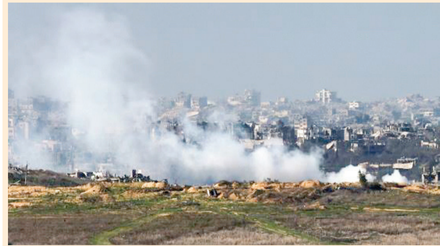
Smoke billows as buildings lie in ruin in Beit Hanoun, in the Gaza Strip, amid the ongoing conflict between Israel and Hamas, as seen from southern Israel, January 8, 2025. Source: Agency
